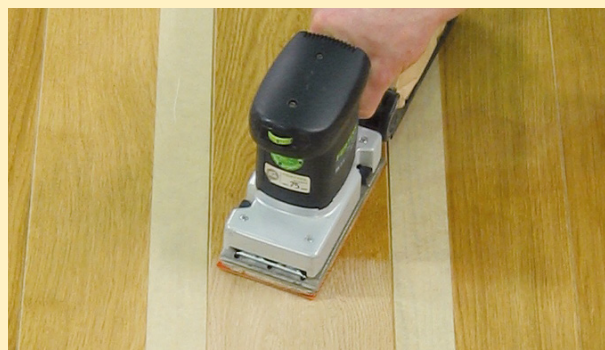
Sand the damaged surface thoroughly.
