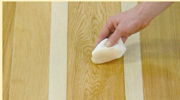
After drying, apply the 2nd coat very thinly with a lint-free cloth.
